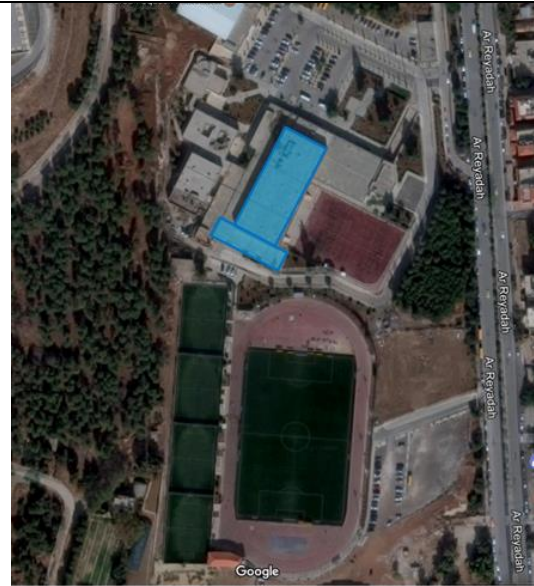
Figure 1B: Location of the UoJ's Sports City Campus, Amman, Capital of Jordan (Blue Boxes identifies suggested rooftop area to be utilized)
